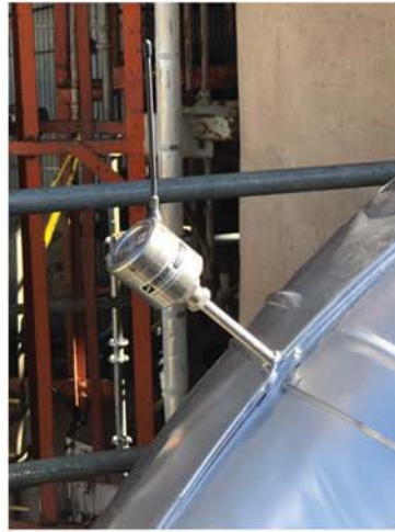
High-temp dual-element unit installed under insulation.
